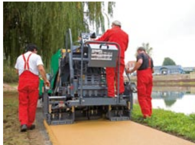
Landscaping and sidewalks
