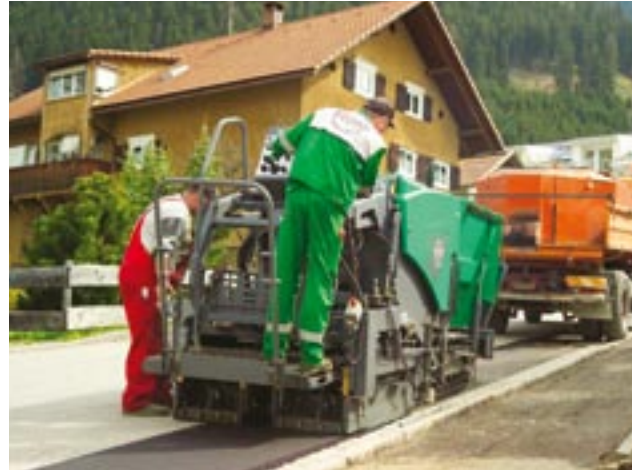
Utility and repair paving
