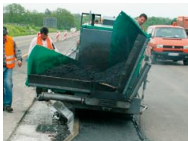
Paving medians, shoulders and road widening
