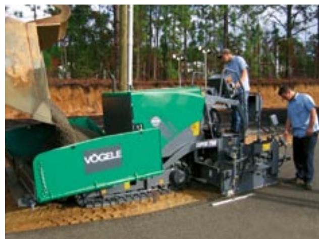
Surfacing traffic areas and roads
