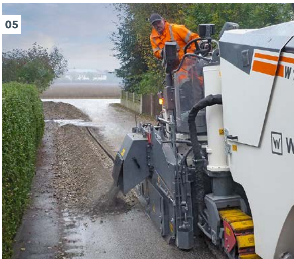
05 To install fiberoptic cables, deep and narrow slots are milled into the asphalt with the deep milling unit.
